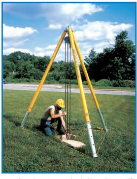
A worker using a Spanco Tripod with Mud Feet to lift a manhole cover single-handedly.
